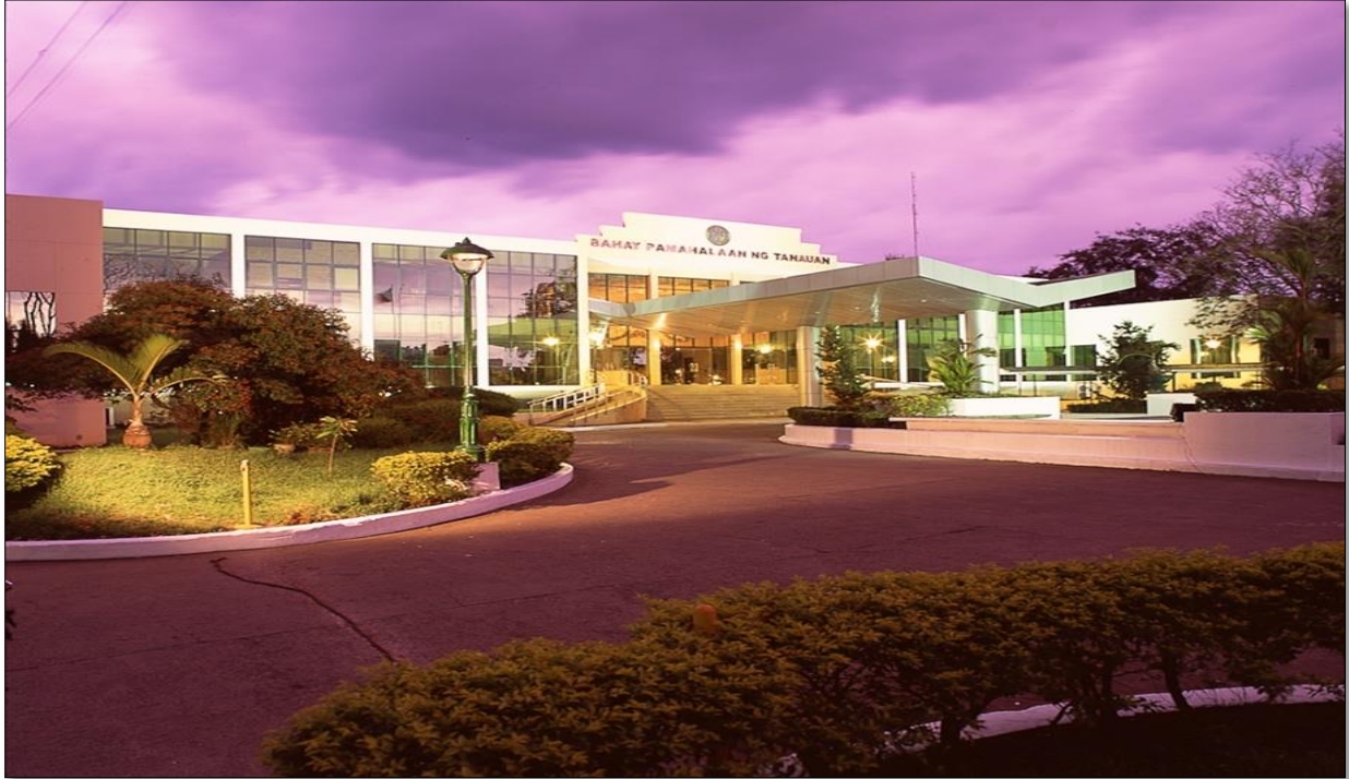
Figure 10. (Tanauan City Hall Executive Building)
